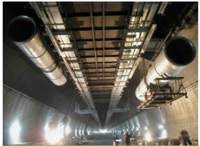
Fig.11. Tunnel ventilation system
