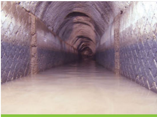
Fig.2. Inside a tunnel
