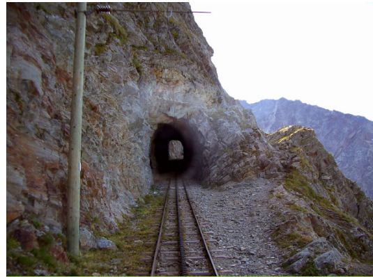
Fig.4. Outside a tunnel
