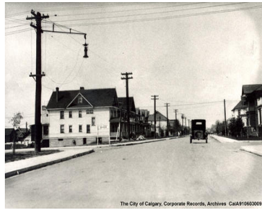
Fig. 4. Carbon arc street light located near Victoria Park
