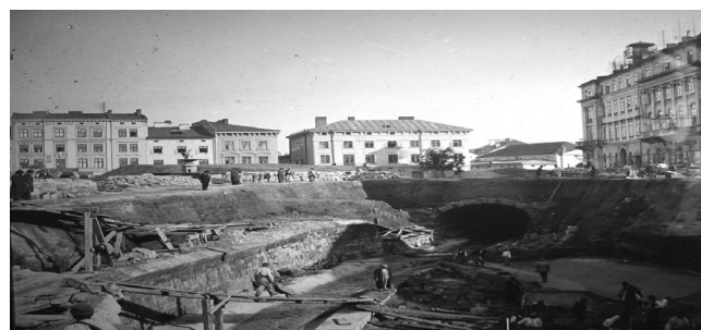
Fig. 3. The overlap of the Poltva river in an underground reservoir
