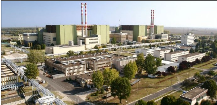
Fig 1 General view of the nuclear power plant of Paks, Hungary
