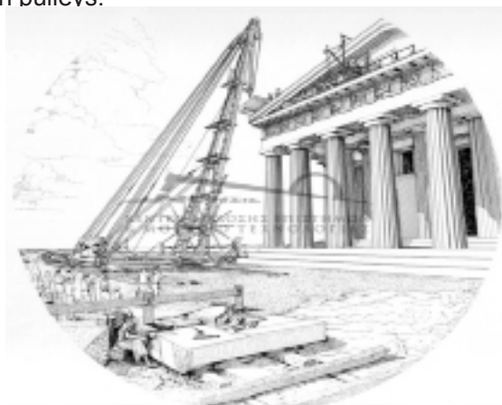
Figure 3: The same rock, using winch elevated to the roof of Parthenon (last page).
